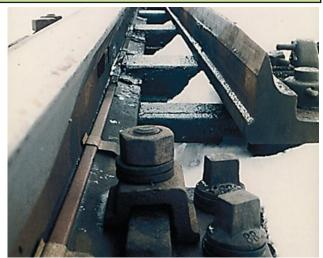
Figure 2: Railway switch equipped with electrical heater. Source: railway-technology com
