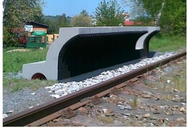
Also, prototype parts of rail noise absorber called BRENS ABSORBER were made in order to increase sound absorption of the rails. Laboratory measurements of noise attenuation were taken. Noise reduction achieved in the laboratory for the whole system was of 14 dB. Results for the barrier alone are not known.
