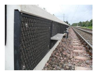
Figure 15 (left): Zbloc barrier. Figure 16: Steps for emergency exit.
